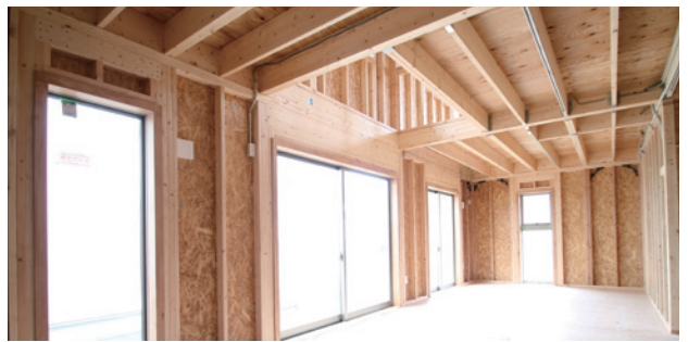
The 2×4 construction is strong on 6 sides.
